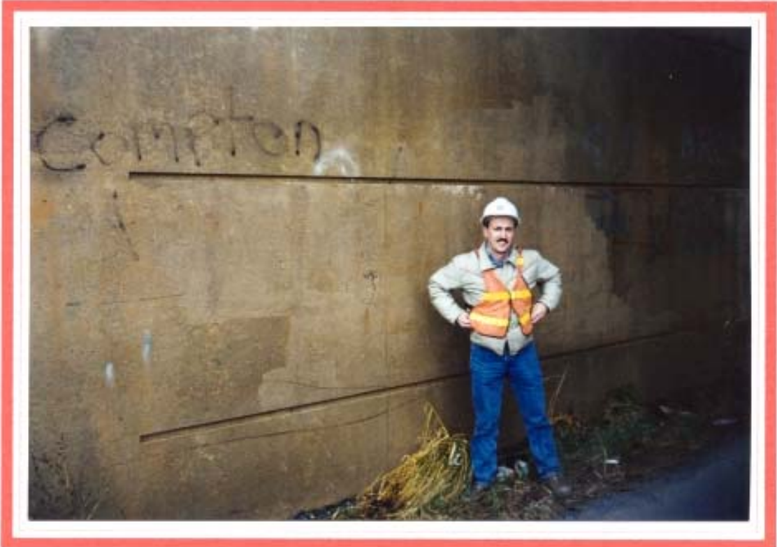
TAGINATOR® removes spray paint graffiti from concrete underpass. ( York, PA )
