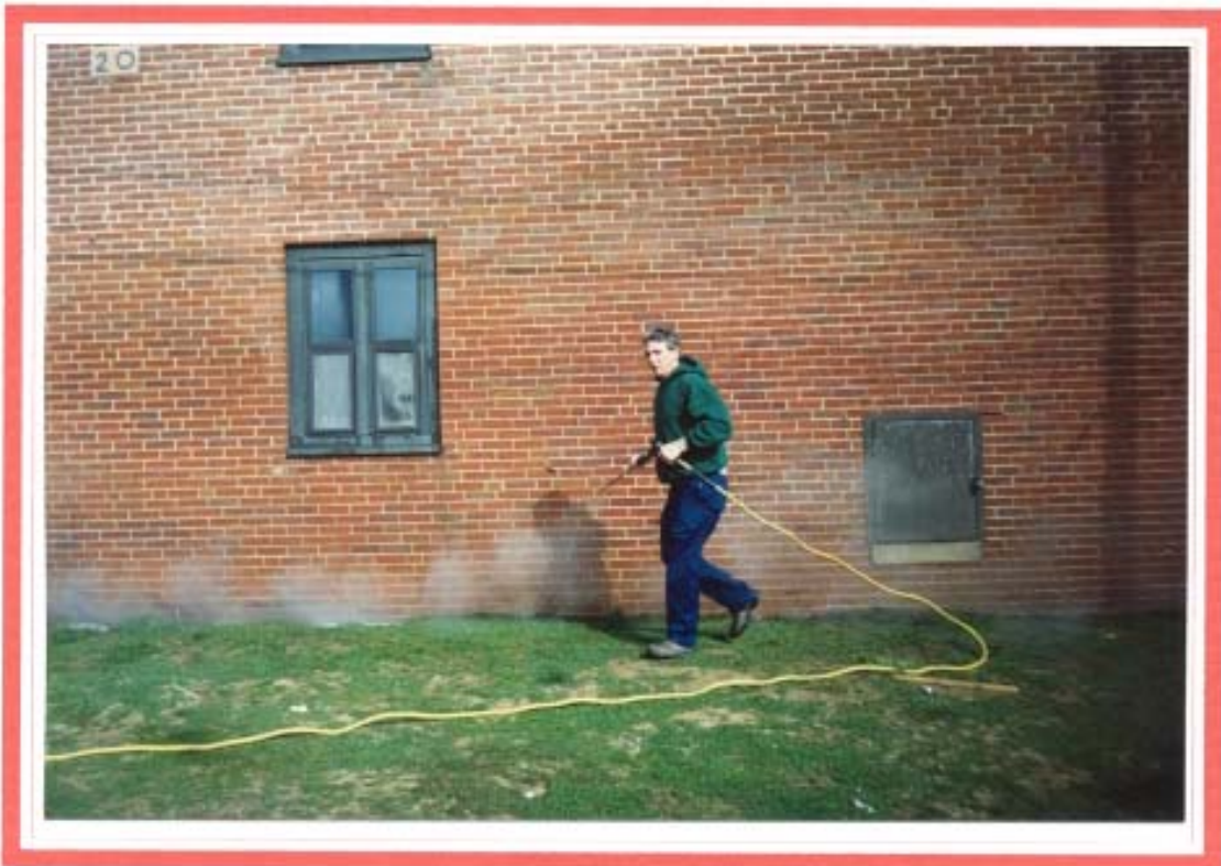
TAGINATOR® removes spray paint graffiti from brick wall. ( Harrisburg, PA )
