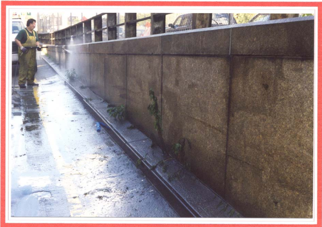
TAGINATOR® removes spray paint graffiti from porous concrete. ( New York, NY )
