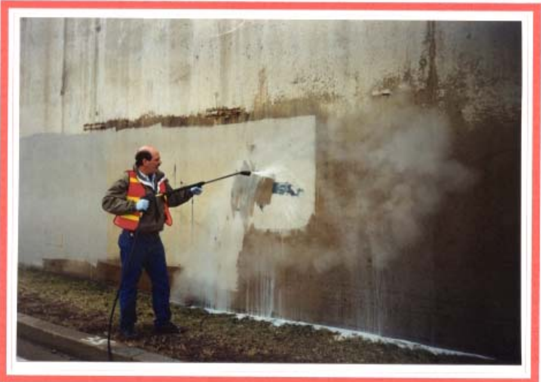
TAGINATOR® removes painted over graffiti from poured concrete. ( Pittsburgh, PA )
