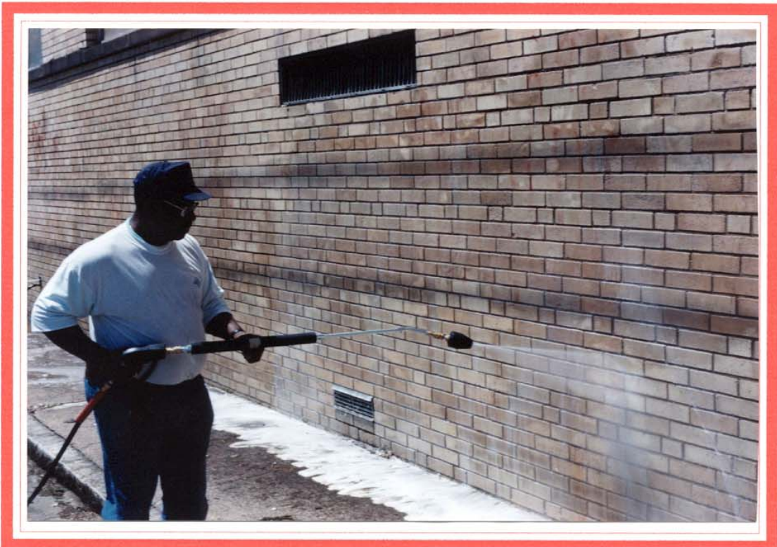
TAGINATOR ® removes red spray paint graffiti from brick wall. ( Harrisburg, PA )
