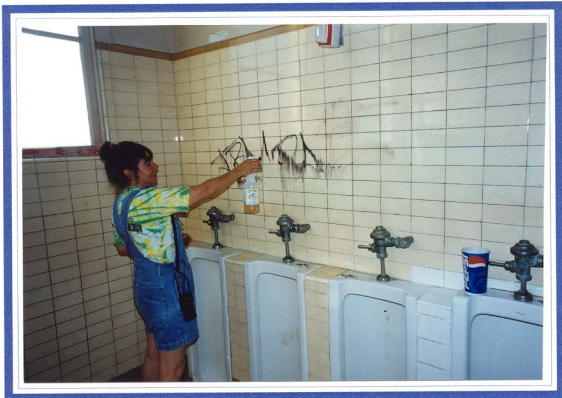
TAGAWAY® removes permanent marker graffiti from ceramic tile. ( Fresno, CA )
