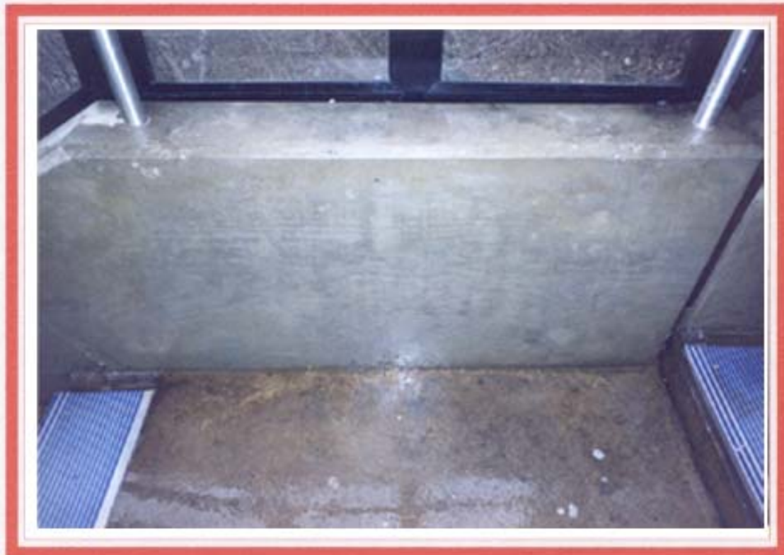
TAGINATOR® removes spray paint graffiti from poured concrete. ( NJ Transit )
