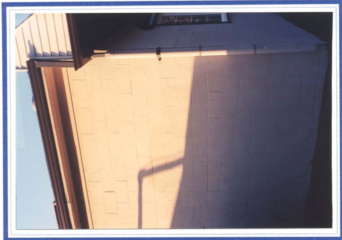
TAGAWAY® removes spray paint graffiti from painted wall. ( Delco, PA )
