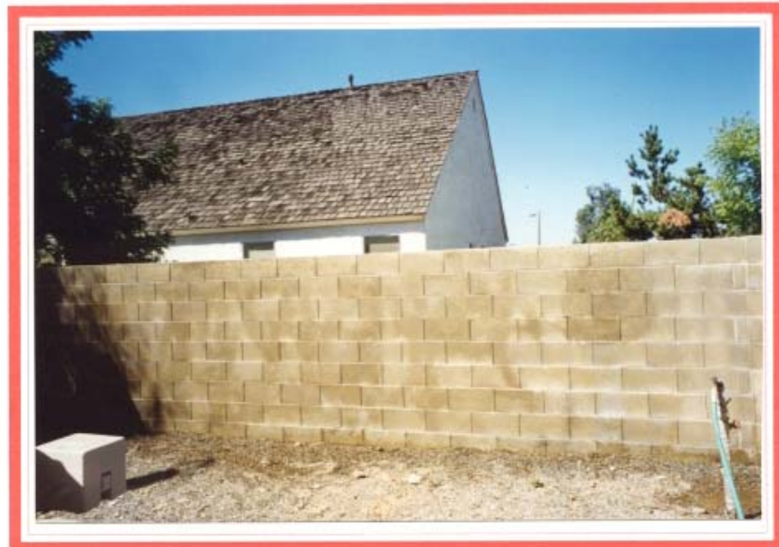
TAGINATOR ® removes spray paint graffiti from concrete wall. ( Fresno, CA )
