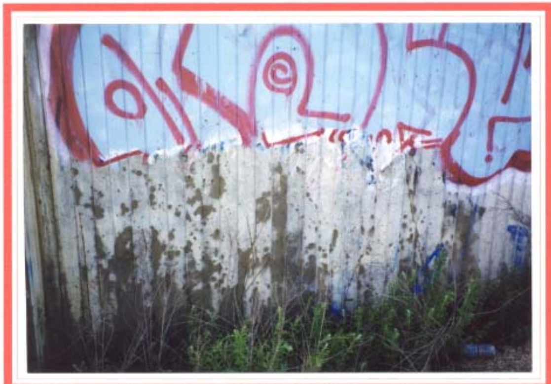
TAGINATOR® removes multi-layered spray paint graffiti from cast concrete. ( Washington, DC )
