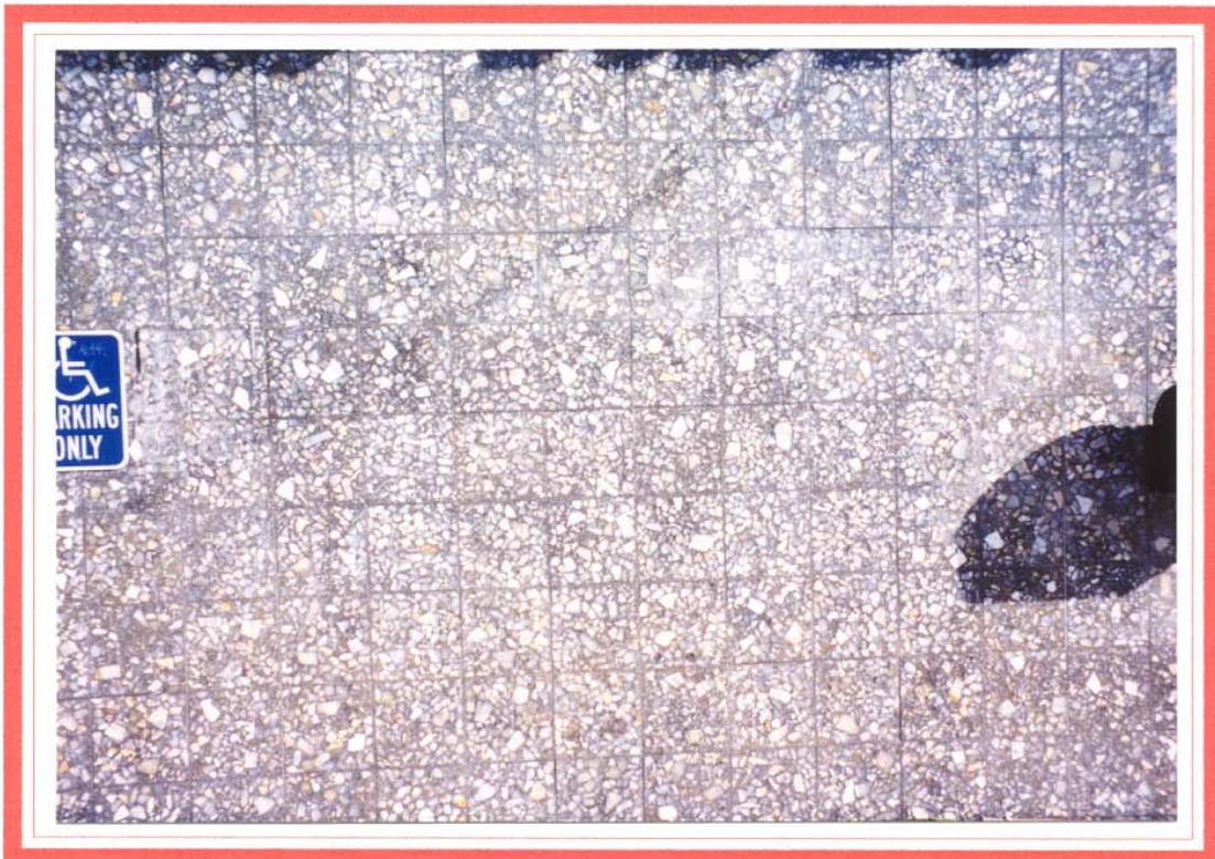
TAGINATOR® removes spray paint graffiti from Terrazzo marble. ( Santa Clara, CA )
