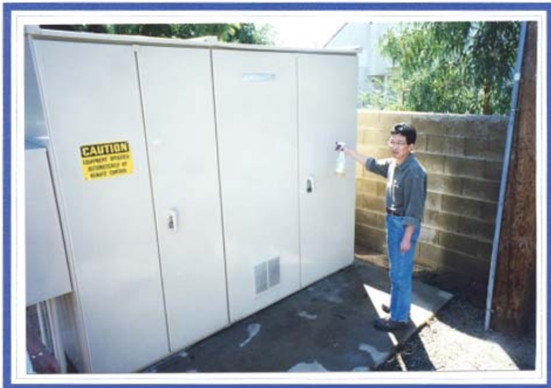
TAGAWAY® removes permanent marker graffiti from aluminum electrical box. ( Fresno, CA )
